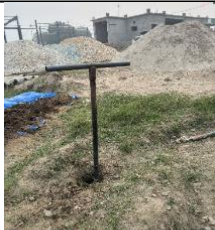
View of Auger placement for Soil Testing
